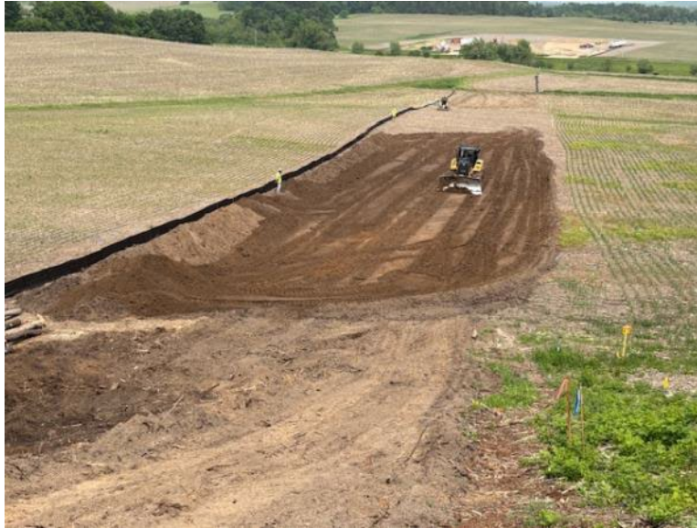
Facing east near MP 3.2, contractor continues topsoil segregation
