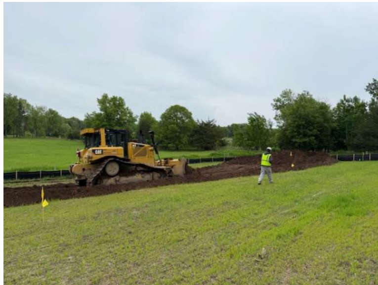
Facing west near MP 1.4, topsoil segregation being completed
