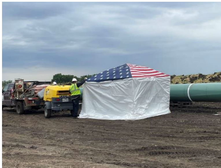
Facing southwest at MP 33.9, K&K sandblasting and coating completed mainline welds
