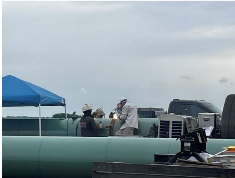
Facing east at MP 33.0, K&K welding mainline pipe
