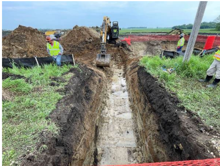
Facing north at MP 34.2, K&K trenching for 165th Street road crossing
