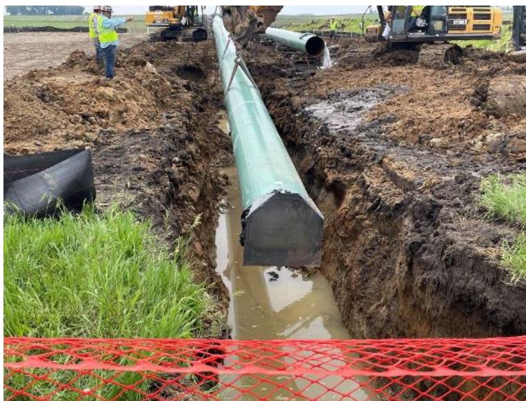
Facing south at MP 34.2, K&K lowering-in four-joint section for 165th Street road crossing
