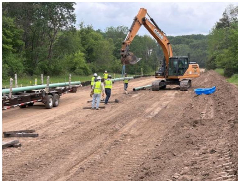
Facing east near MP 2.7, contractor stringing mainline pipe
