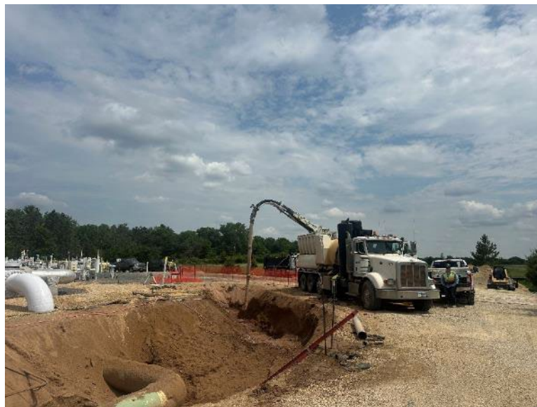
Facing east at MP 0.1, view of Otis utilizing the hydro vac truck in the Hugo compressor station
