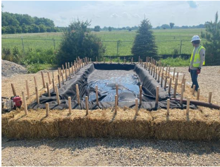
Facing south at MP 0.1, view of the dewatering structure in the Hugo compressor station
