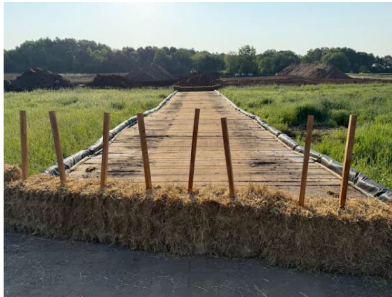
Mat crossing of wetland ERT-W15 completed
