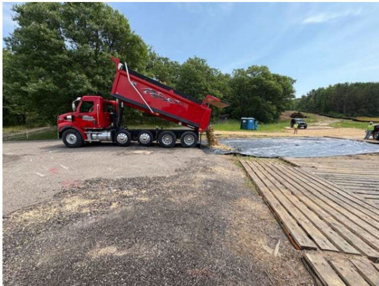
Facing east near MP 2.25, contractor installing tracking pad
