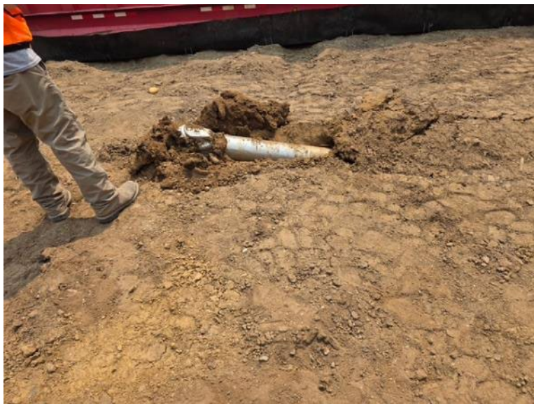
HDD P4-3 completed pilot pass and commenced ream pass
